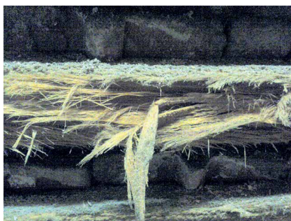
Abb. 6: Mazeration an Dachlatten
